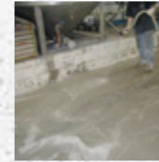
Cleaning/ rinsing surface from debris.
