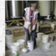
Mixing AQUAFIN ASODUR®SG2 in supplied container.
