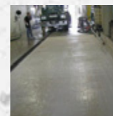
Finished surface, ready to receive top-coating.
